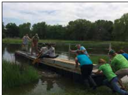
Staff installing a new floating bridge at the pond.
